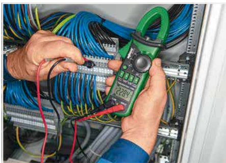
Current measurement in a control cabinet
