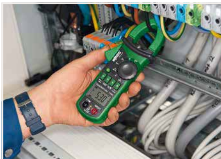
Voltage testing in control cabinet
